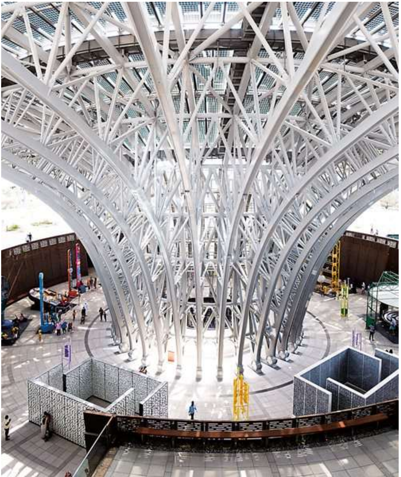
Inside Terra, the roof's "eye" of sloping, ribbed steel descends to a courtyard and creates a natural vent to let heat rise out of the building.
